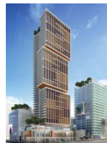
Telus Garden, Vancouver Will be built to LEED Gold Standard
